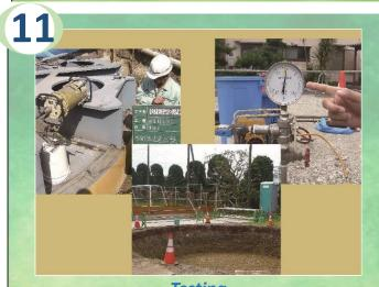
**Testing**Perform each necessary testing, welding inspections, pressure test, water infiltration test, water quality tests.
